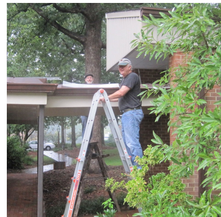
Mike Taylor and Charlie Fetter installing gutter guards.
